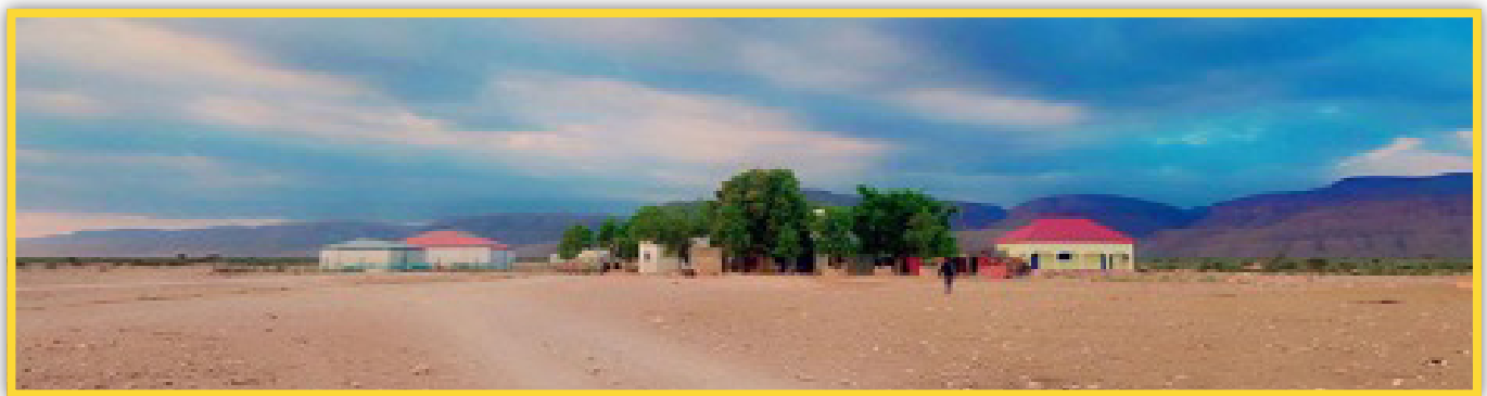
The Main Water Storage Facility of Ufeyn District
